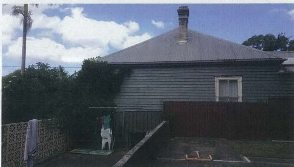
Figure 20: Detail of western elevation of the main hipped roofed section of the house, with chimney. Note timber-framed double hung window with vertical glazing bar to each sash.
