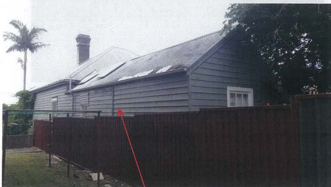
Figure 22: Detail of the western elevation of the house and the gable roofed rear wing from Belmore Lane at the rear. The point at which the pre-1949 extension of this wing starts is arrowed.
