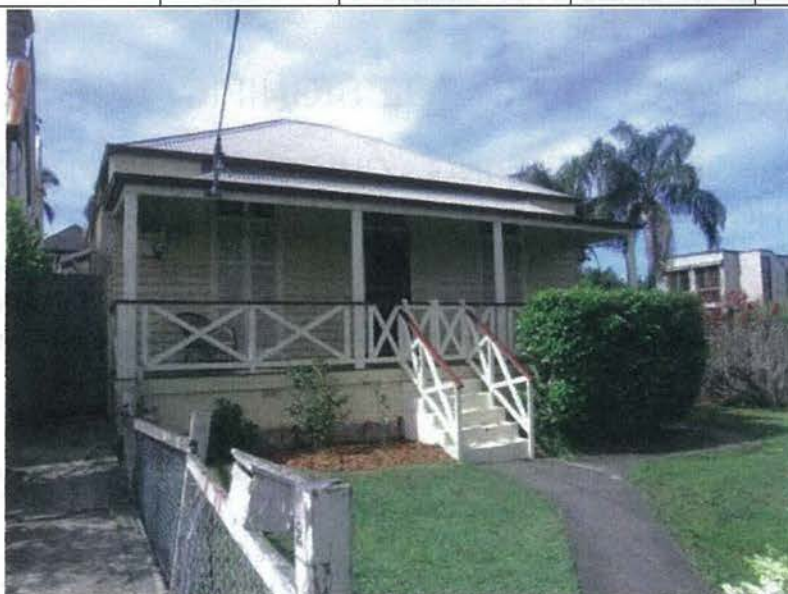
Figure 31: 1868 weatherboard cottage at 2 York Crescent, Petersham Source: State Heritage Inventory form
