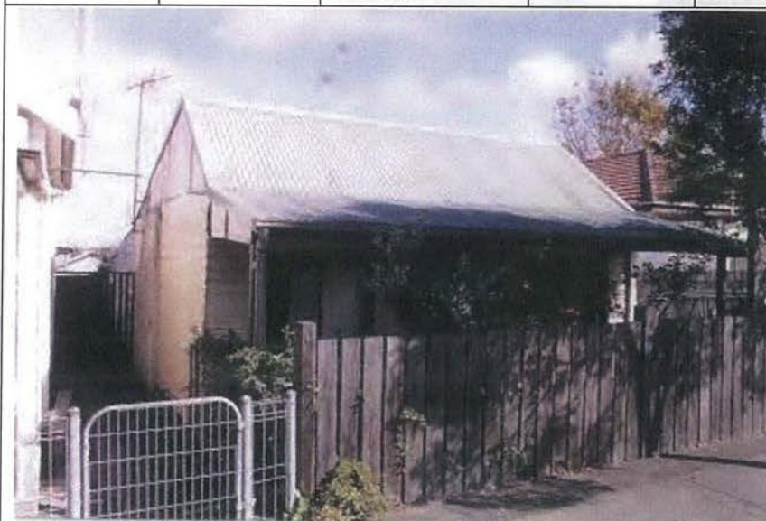
Figure 32: Circa 1940 Timber slab cottage at 44 Barden Street, Tempe. Source: State heritage inventory form
