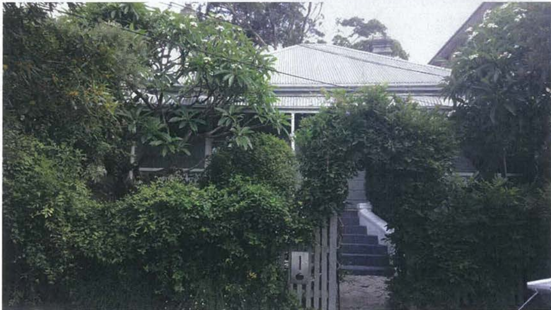
Figure 16: Detail of the front (north) elevation of the house at 34 Belmore Street, Enmore, as seen from Belmore Street. Cast iron verandah posts and balustrade and verandah roof can be seen.
