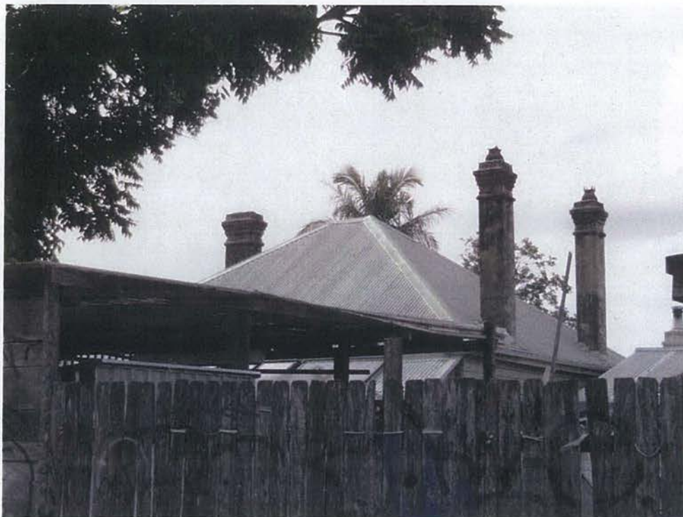
Figure 25: Detail view from Belmore Lane to the east, showing the main roof with all three chimneys, and rear shed structure.
